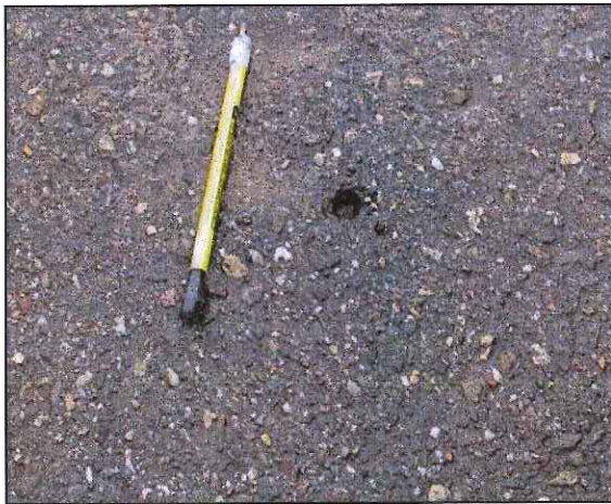
DRILL 1/2" HOLE THROUGH PAVEMENT AND/OR ROADBASE TO ALLOW CONNECTION TO SOILS.
